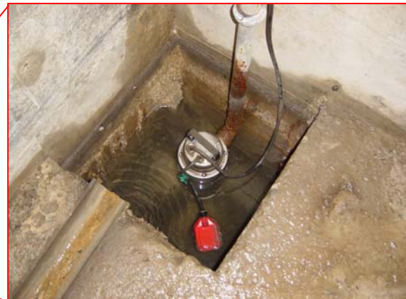
Abb.17: Pumpensumpf
